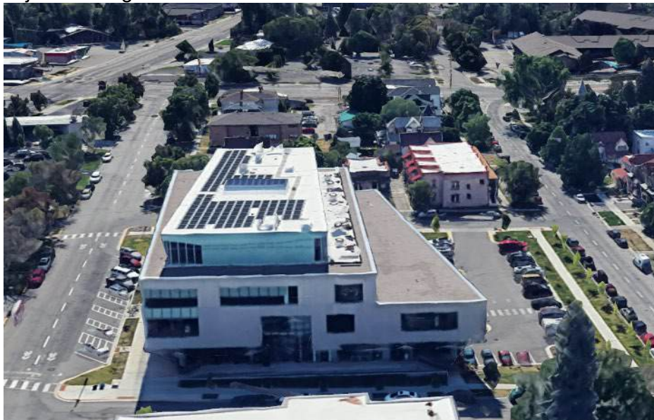
Figure 1: Missoula Public Library – 2nd and 3rd level rock ballast roof
