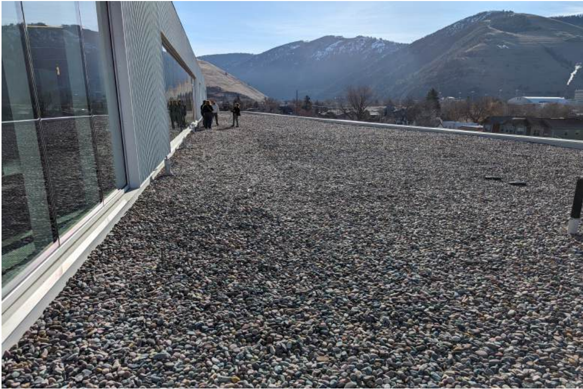
LEVEL 2 ROCK BALLAST ROOF
