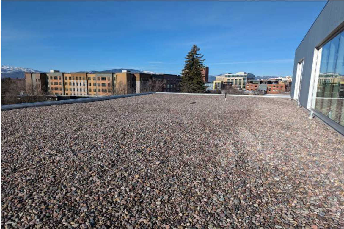
LEVEL 2 ROCK BALLAST ROOF
